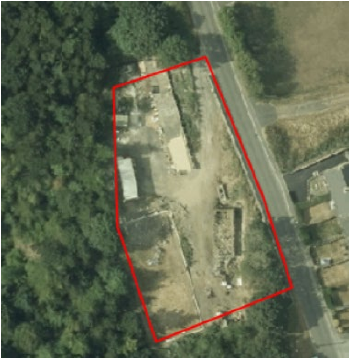
Figure 2 - aerial of the site in 2018
